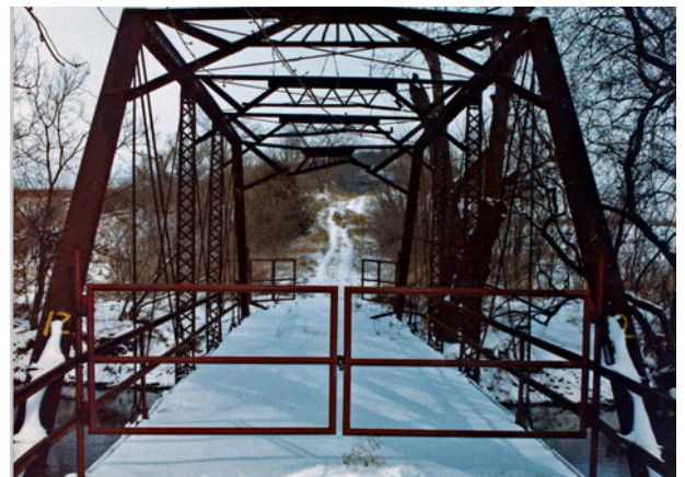
Bridge 12 - Jug Creek
