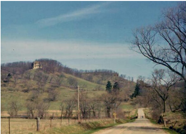
View of Blackhawk Rock and Bridge 13
