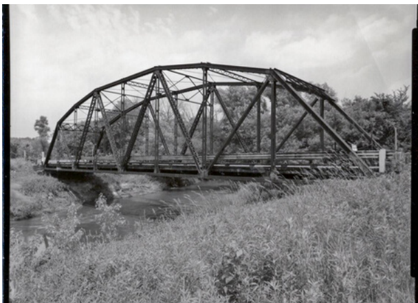
Bridge 18 - Bacon's Bridge
